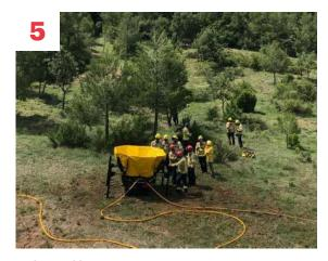
**Tank assembly**A light structure for easy water tank deployment and assembly.
