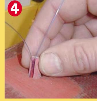
Remove the bars and ensure that the injury is in the centre of the clamp. The bars are not needed anymore. Squeeze the hose to open it. Fold the nylon line keeping both ends of the nylon folded back (see above), and push the internal plug patch into the hose and align as shown. Reclamp the hose, centrally. Leave the nylon in place
